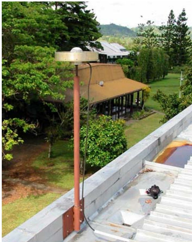
Figure 3. LAE1 IGS Reference Station on the roof of the Sandover Building, DSLS, UniTech
