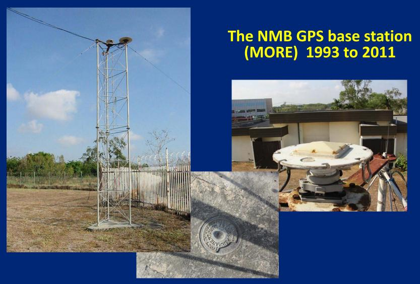
Primary GPS base station for PNG Geodetic surveys Used in development of PNG94
